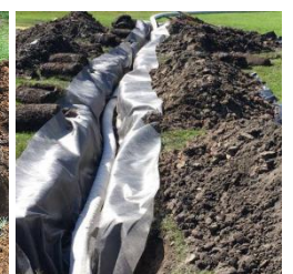
French Drain to Dry well
